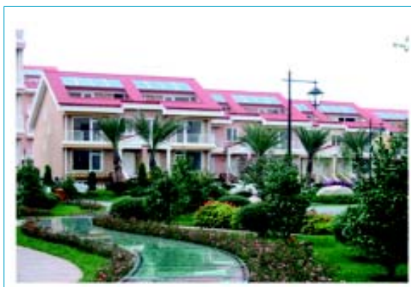
Figure 4.3 Solar water-heating system for building in Kunming city, Yunnan Province
